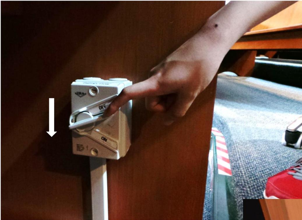
**4. Turn on the power switch under the desk for the operating console.**
